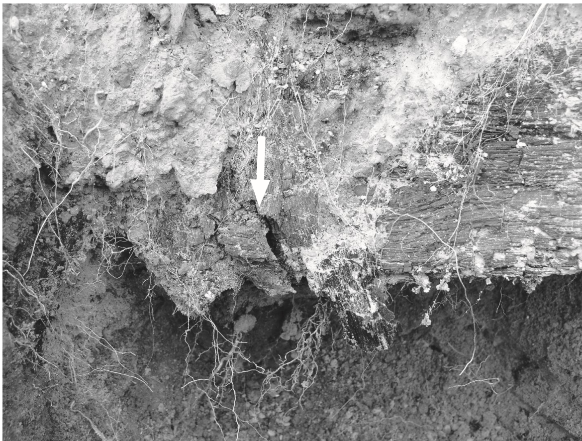
Fig. 2. Beams 2/2008 and 3/2008 joined perpendicularly by an iron nail (see arrow).
